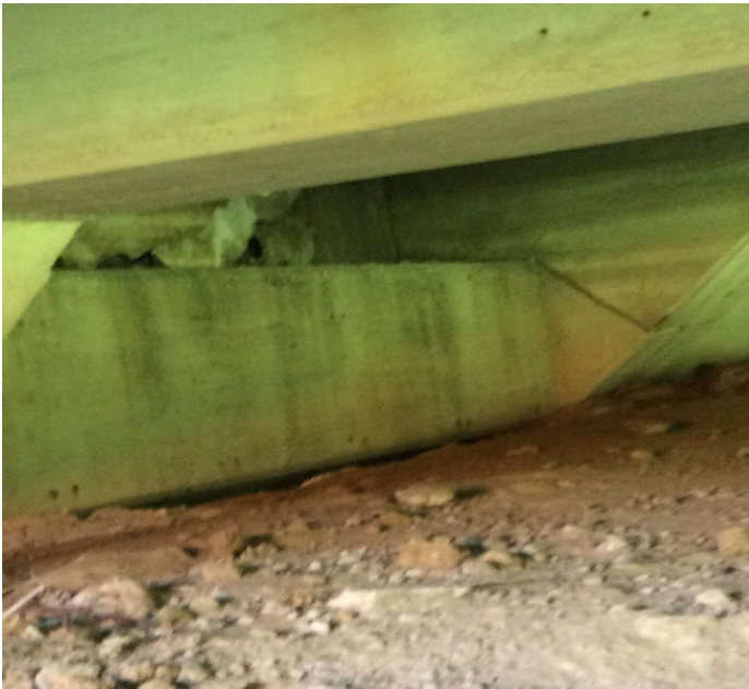
PHOTO 1 Description Large slab spall w/t efflorescence & rust stains to backwall between girders 2 & 3 at Abutment 2.
